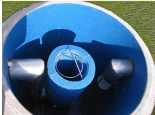
Since the inside of the separator should be periodically inspected and cleaned, it is advisable to locate the unit outside any roads, parking lots, etc. Location of the unit should allow easy access of the vacuum trucks for performance of maintenance work.
